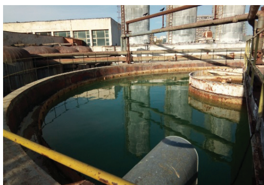
(a) View with lime tins, mechanical filters and primary radial settling tank
