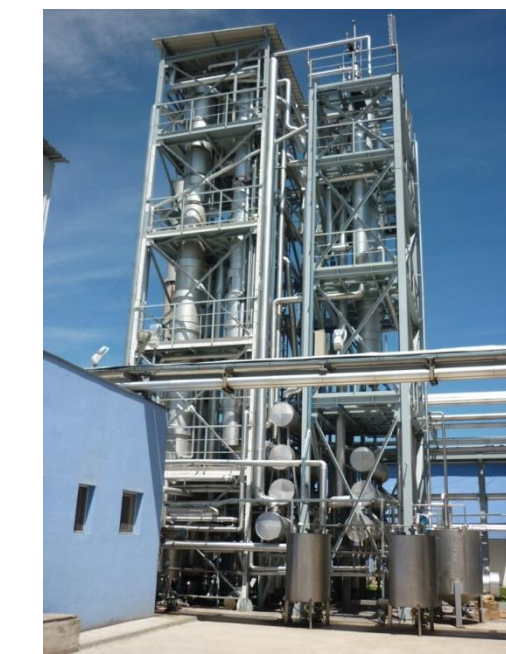
Four column rectification plant for high quality ethanol > 96.3% ; Productivity 20 000 l/day.
